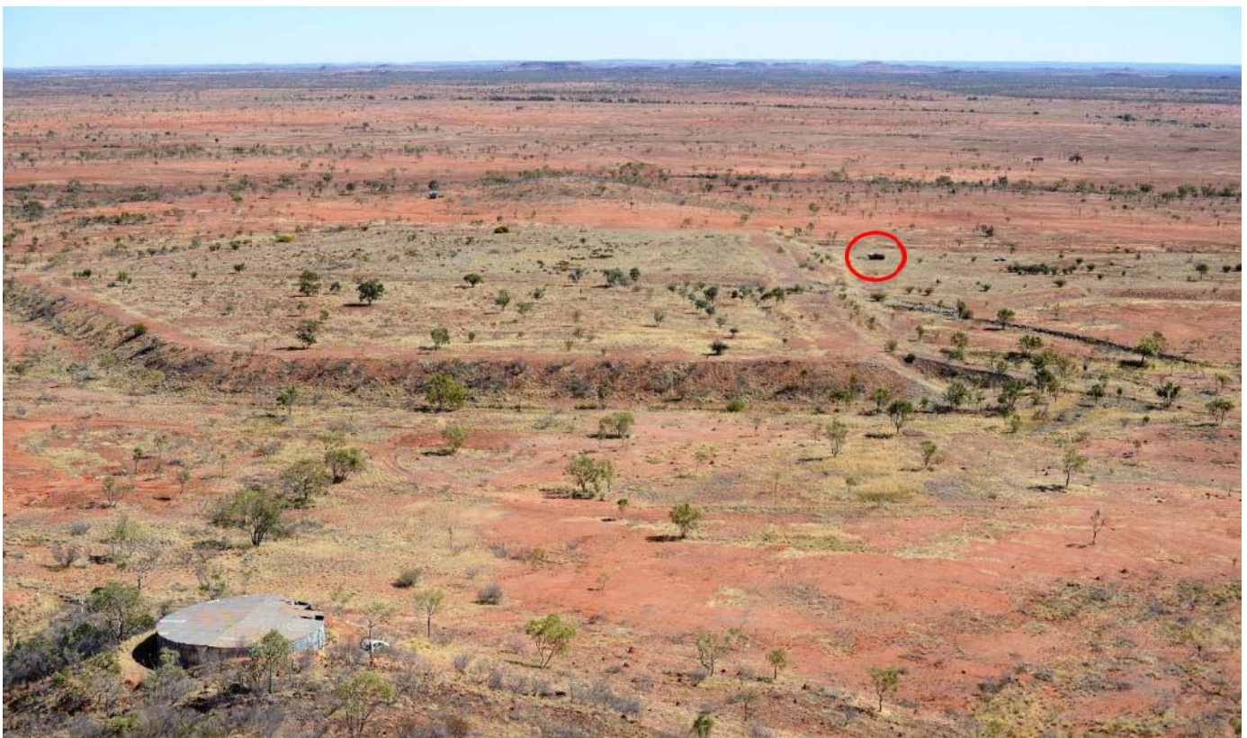
Tick Hill Tailings Dam, looking west over the water storage tank from the flank of Tick Hill. Drill rig on decant pond circled in red
