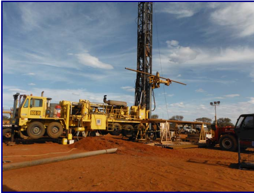
Cyclone Project – Water Bore drilling rig loading a 9m drill rod
